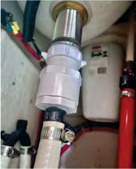
New sink drain connections
