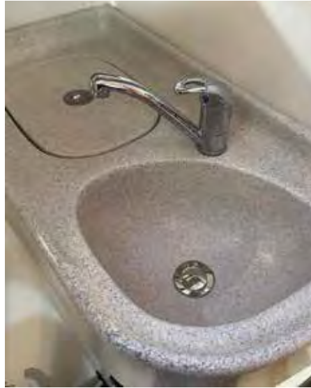
New sink drain install
