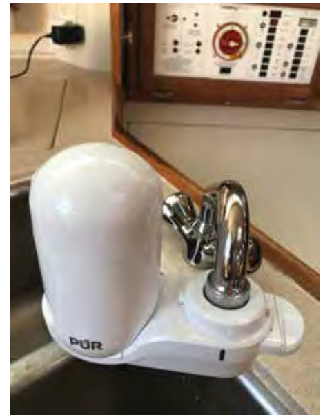
PUR water filter on galley sink faucet. Note small, flat switch at right of filter. In this position, water bypasses filter. Move switch down for water to pass through filter.
