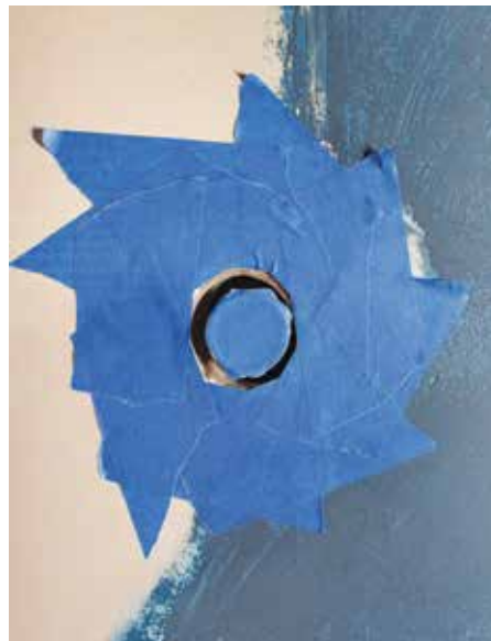
Ready for epoxy
