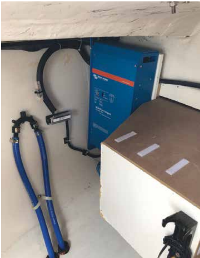
Installed Multiplus
