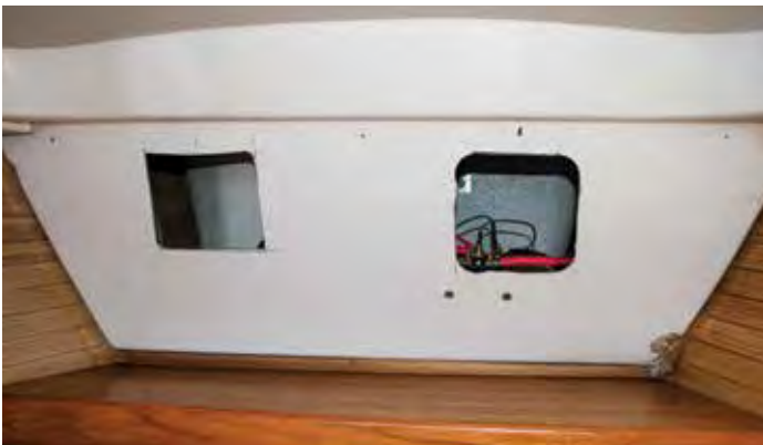
Decorative plywood panel removed and two access holes cut in the hull liner. You can see the top of the solenoid and one of the backing plates in the right hole.
