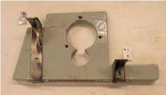
Underside of the shelf with the brackets in place. The small rectangular plates are the backing plates for each bracket.
