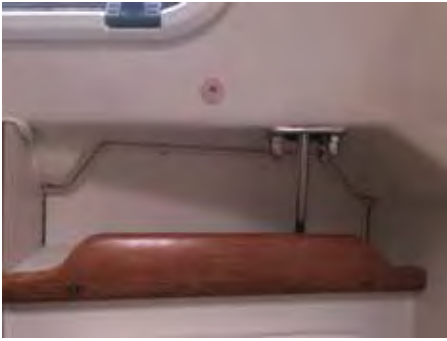
Panel had to be removed to gain access to holding tank.
