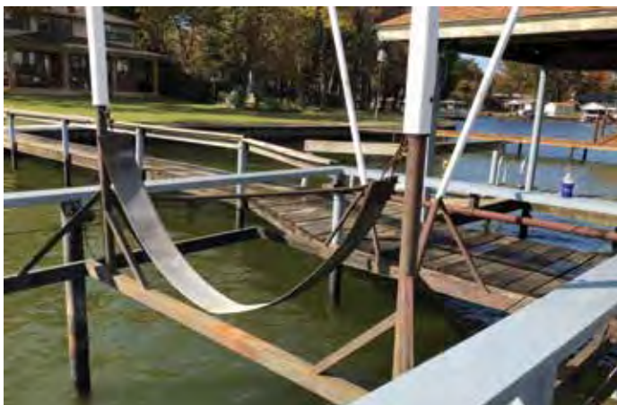
Original lift cradle
