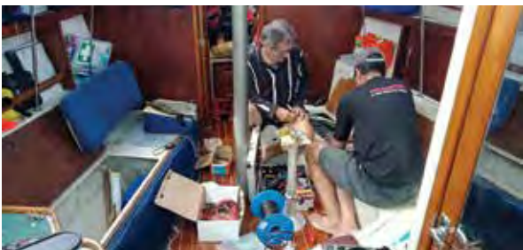
Below in the cabin, lots happening; new batteries, new solar panel and all connections, engine service, checking the charters, new sat phone set up.
