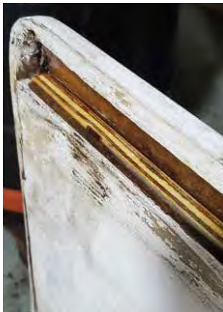
Sealing the edges of the new core
