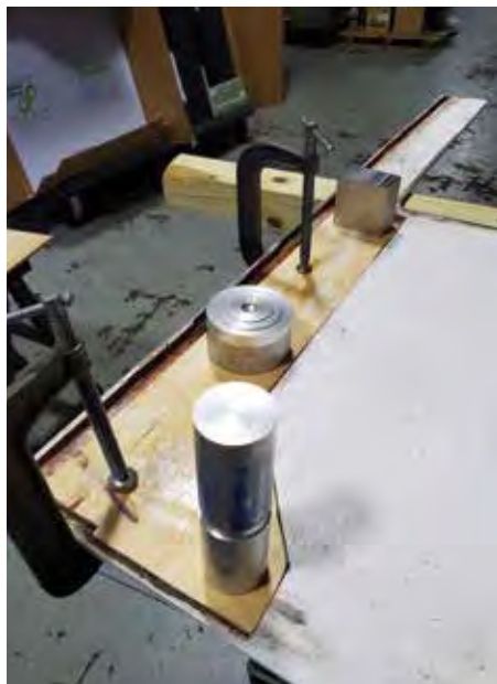
Bonding the new core in place
