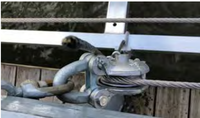
New pulley and cable
