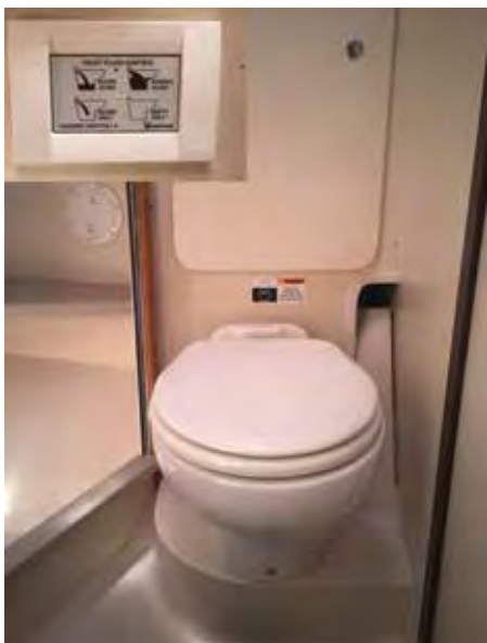
Finished project with optional controller shown in inset which was mounted under vanity sink.
