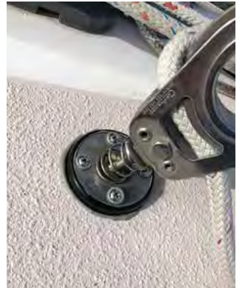
Finished result prior to cleaning excess butyl tape.
