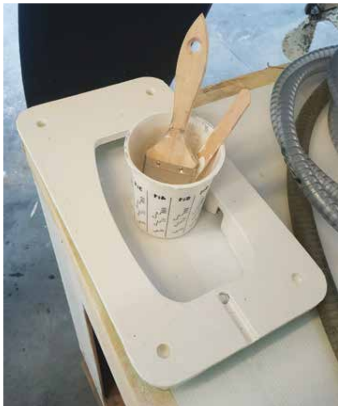
The underside of the new mast step after being coated in Epoxy Flowcoat to prevent dissimilar metal contact.
